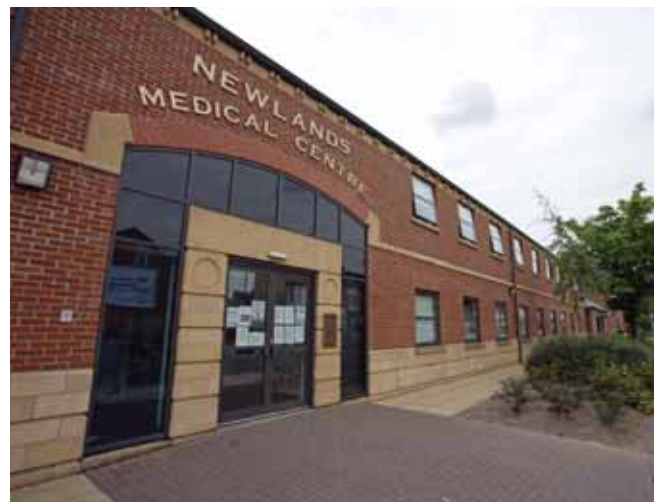
The Newlands Medical Centre, Borough Road
