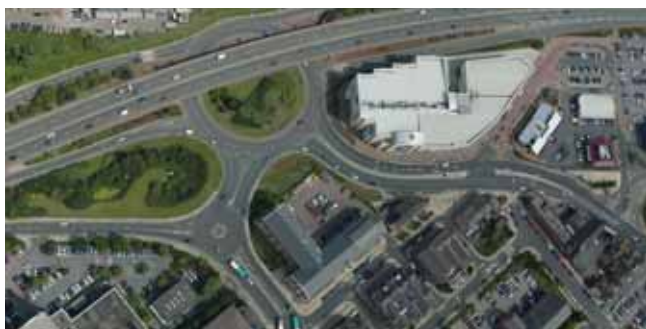
An aerial view of the Marton Road/A66 junction close to Middlesbrough town centre
